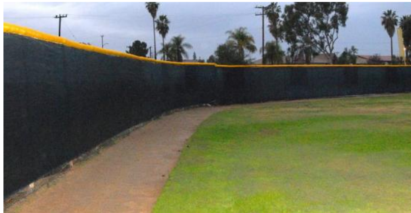
Major Field Warning Track & Protective Fence Tops
